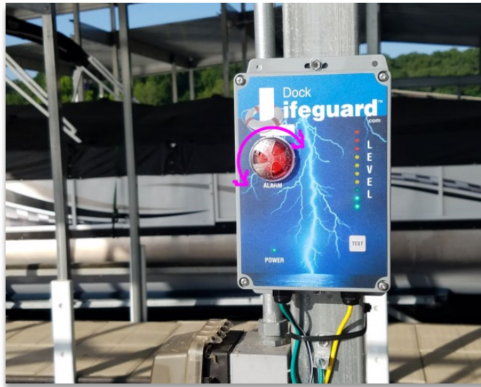
Figure 5, Rotate Clear Ring Over Red Light to change Volume Level
